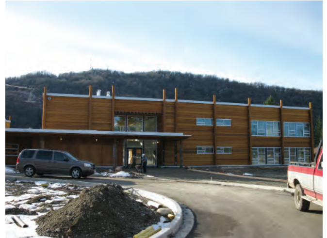
High School Construction 2009
