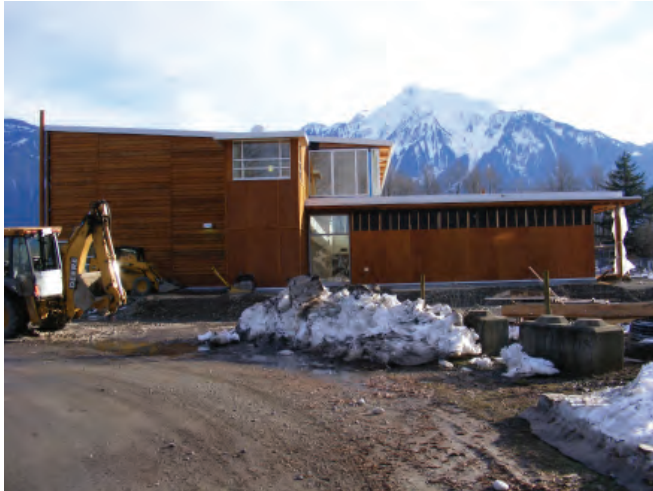
High School Construction 2009
